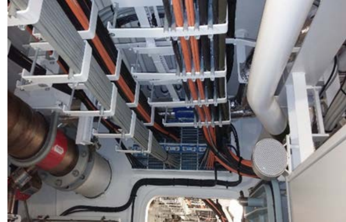
Large Passageway & Cable Trays (StanFlex Frigate Visit in Nov 2014)
